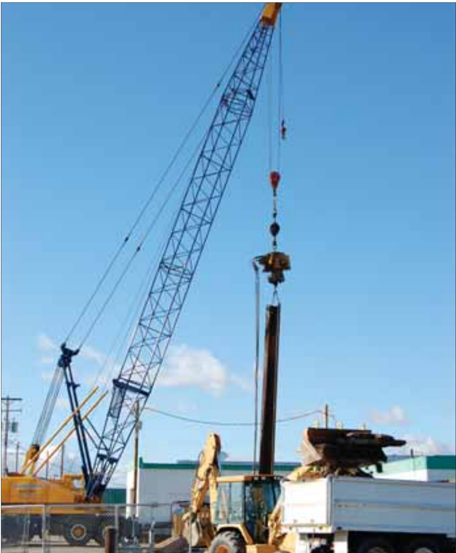
Nampa-based G&S Excavation has been driving large slabs of steel into the ground in preparation of removing storage tanks at the corner of Idaho Avenue and Main Street.
